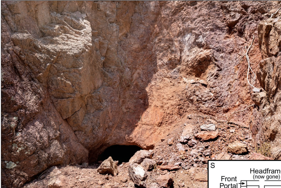
Figure 5. North adit of Ford mine, still partially open in 2019. Christi Cramer photo.
