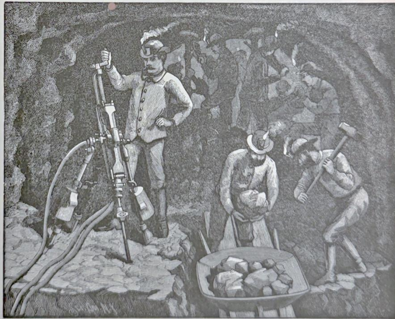
FIG. 148. INGERSOLL DRILLS AT WORK IN A TUNNEL.
