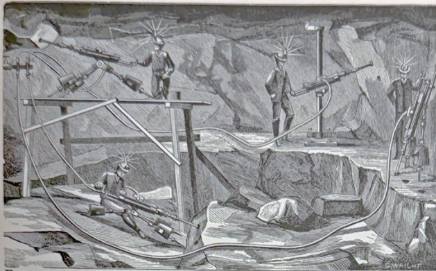
FIG. 147. STOPPING AND PIT MINING WITH INGERSOLL AND SERGEANT DRILLS.
