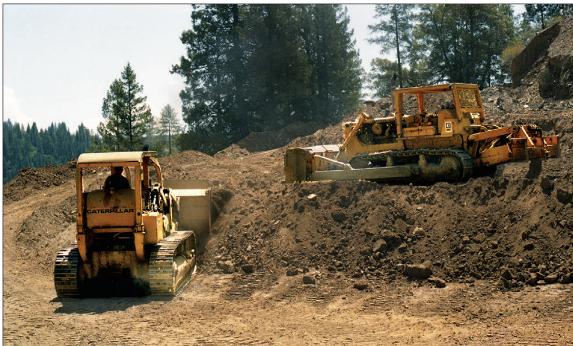
Figure 36. Heavy equipment being used to remove large quantities of rock to expose gold-bearing veins in the Red Ledge mine open pit. Terry Szenics photo, August 2009.
