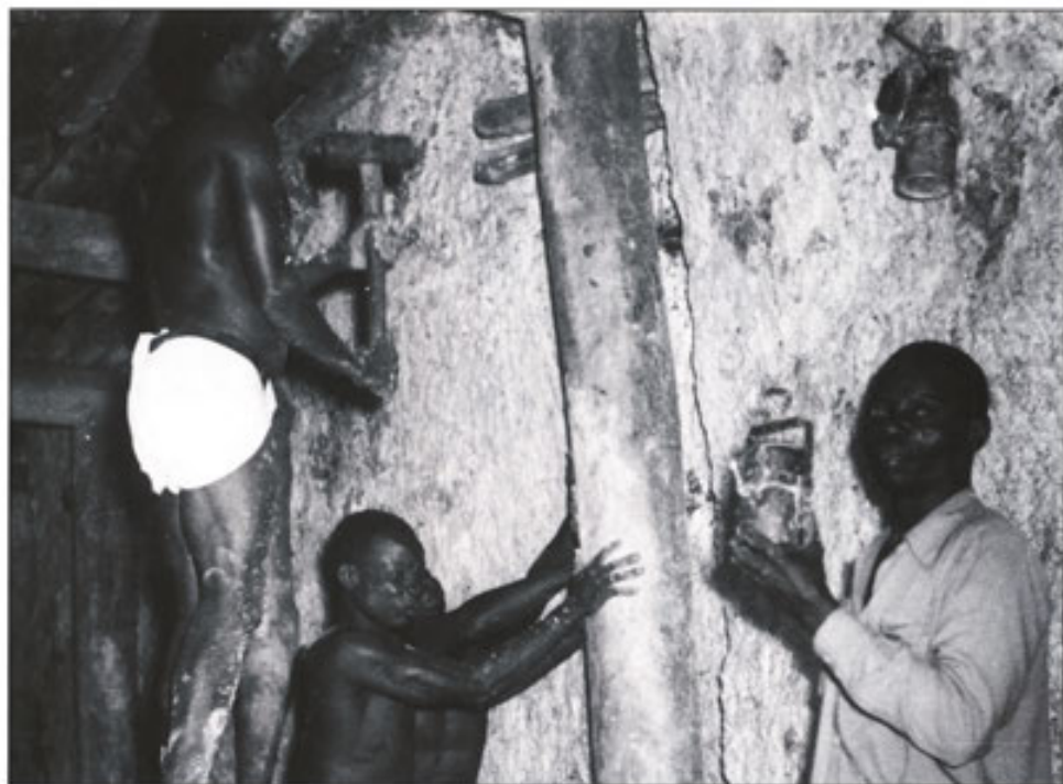
Figure 3. Hammering timbers in place at the Muiane mine ca. 1956. Danilo S. Picolo photo.
