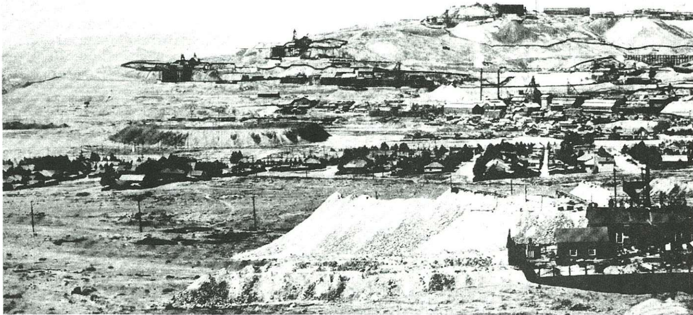
MAIN RANGE SURFACE PLANT LOOKING WEST TOWARD BUTTE HILL
