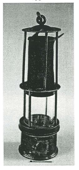
Class of Lamp: Benzine Safety Lamp / Nr. 6 A with special inspection device used for viewing from above when lamp is suspended in pit.
