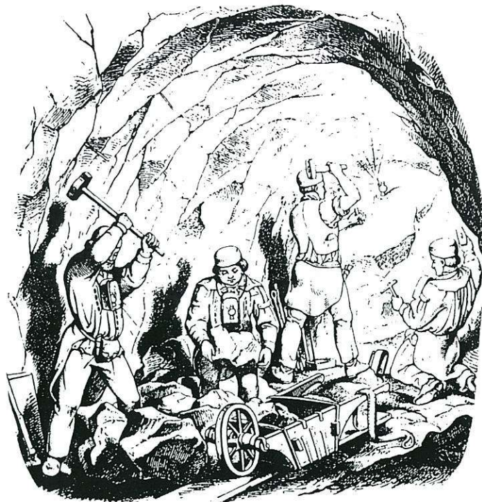
Figure 3. Miners driving a tunnel with only Schlagel and Eisen (hammer and pick). Three are wearing their Blenden on their chest, while a fourth has removed his coo-coo lamp and mounted it on the working face (illustration from Eduard Heuchler's Die Bergknappen in Ihren Berufs- und Familienleben , 1857).
