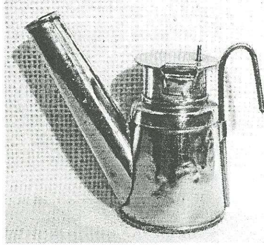
Copper and brass Trethaway Bros. oil wick with brass vent tube located at the rear of the cap. D. Johnson collection.
