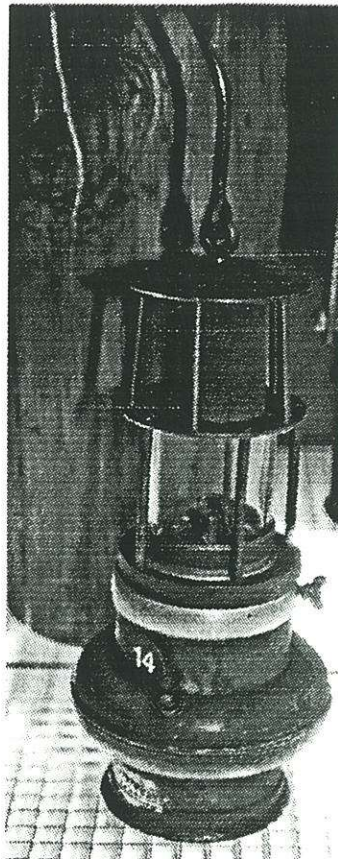
Friemann & Wolf, carbide safety, 1907, inventor: Stuchlik, coal mining in Bavaria.
