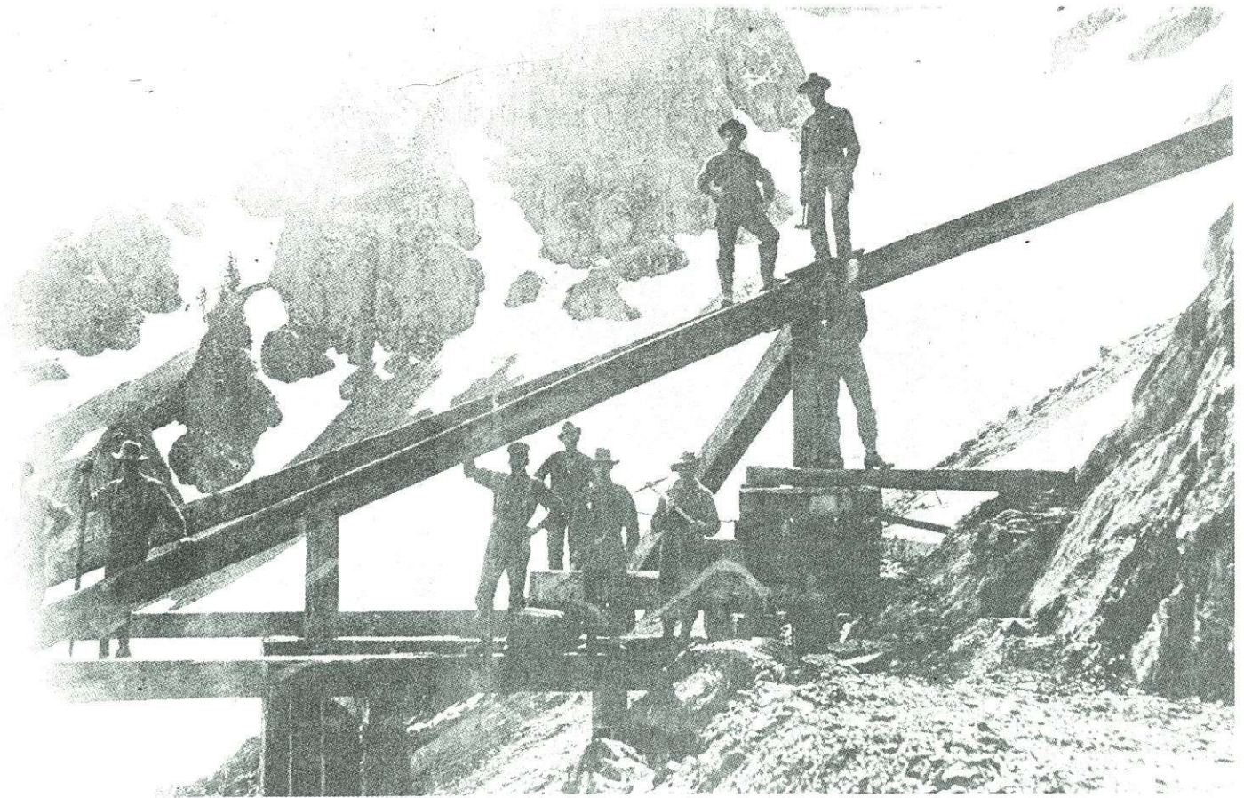
Rebuilding the Stampmill near the mouth of the mine tunnel after the fire.
