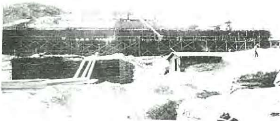
VAT LEACHING, c. 1917. These are the vat leaching tanks that the NCCC constructed to hold the broken oxide ores while they were being leached. Photo from George A. Newett.
