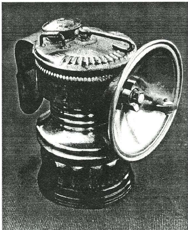
Above: Universal Dropper with spade mount. Lamp borrows Auto-Lite's reflector, wing-nut and Bumper-grip.
