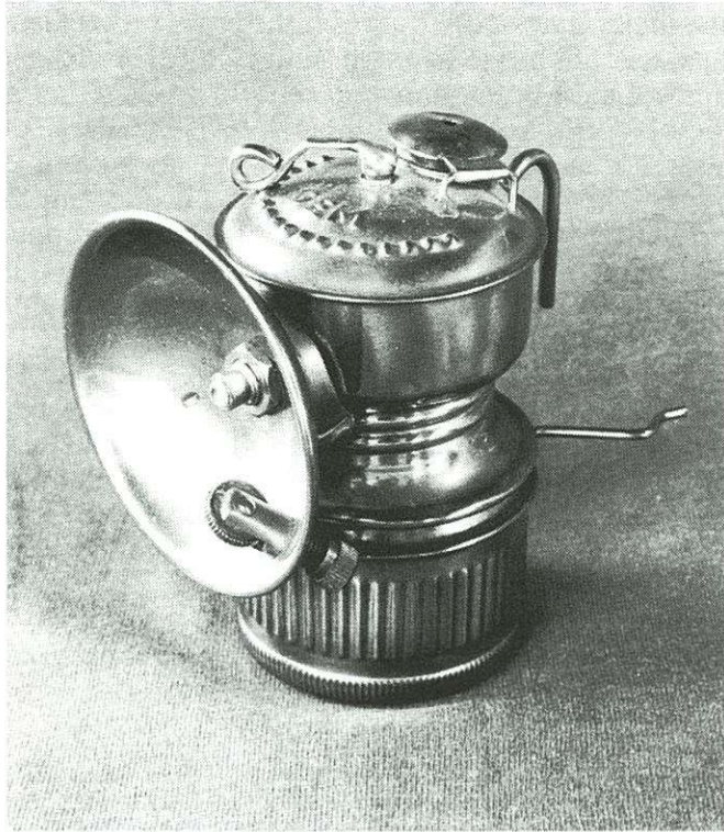
GEM cap lamp, brass, 2 1/2" reflector.
