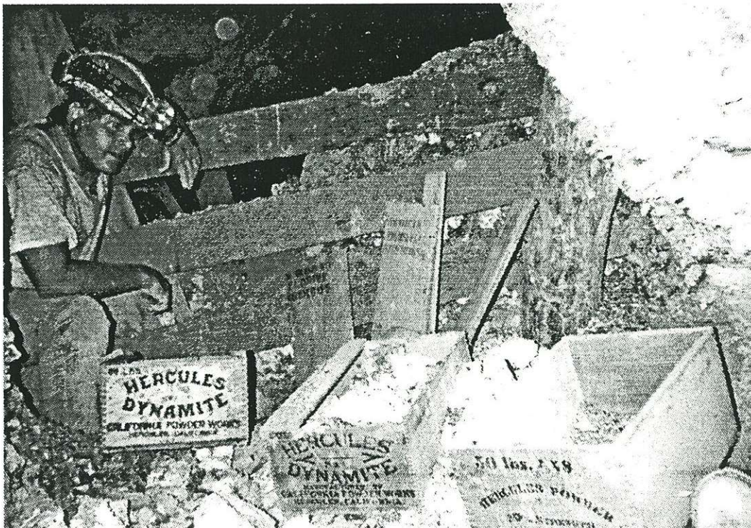
One level was loaded with dynamite boxes.
