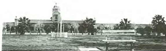
THE PLAZA, c. 1923. Complete with Flag pole, it was the only grassy plot of ground in the 300 miles between Tucson and Yuma. Photo from George A. Newett.
