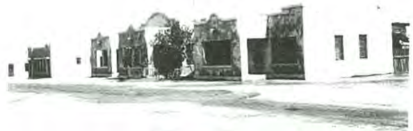
AJO HOUSES, c. 1920 This image of the Ajo housing was made by George A. Newett during a New Cornelia Copper Company Board of Directors meeting at the mine some time in the early 1920's. Apparently these are duplex houses in what was called Mexican town. Photo from George A. Newett.
