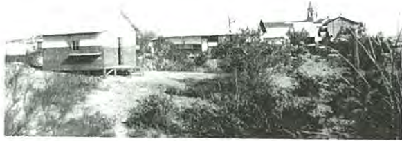
EARLY AJO HOUSING, c. 1917. The tent house on the left was typical of about 50% of the housing in Arizona at the turn of the century. One of the NCCC's first activities was to provide adequate housing for all of its employees. In spite of the best efforts of the company some of these tent houses remained in Ajo until the late 1940's. M. Curley School in the background. Photo from George A. Newett.
