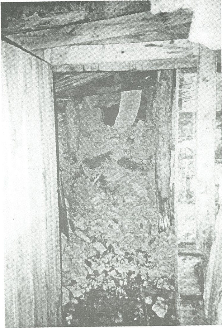
Mines of this type are not a good thing.
