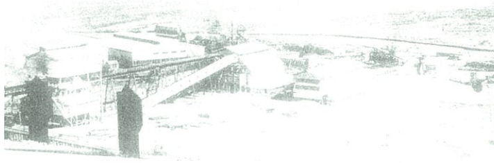
THE MILL AT AJO c. 1923. An overall view of the mill. The smoke stack at the left was from the sulfide roasting plant which roasted ores from Bisbee to provide sulfur gasses for the leaching operation.
