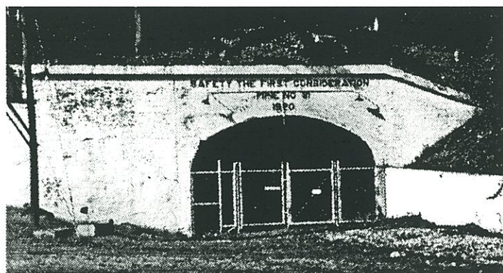
Mine Portal. Lynch, Kentucky.
