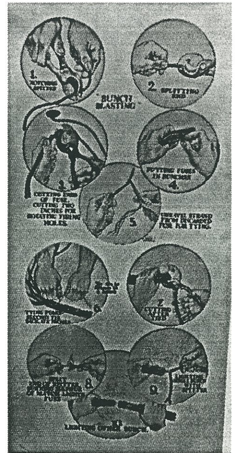
Fig. 4. Bunch Blasting using PEXTO fuse cutter.
