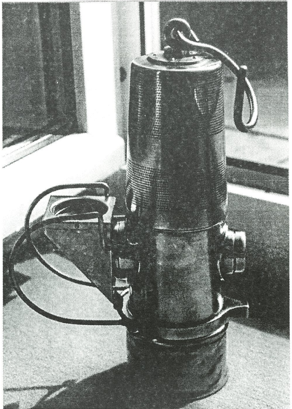
"Singing" Wolf-Fleissner safety lamp No. 713a. Order code was: sigma, 1925. Lamp is fitted with screw lock, two lenses, and prismatic mirror. Height: 30.0 cm.
