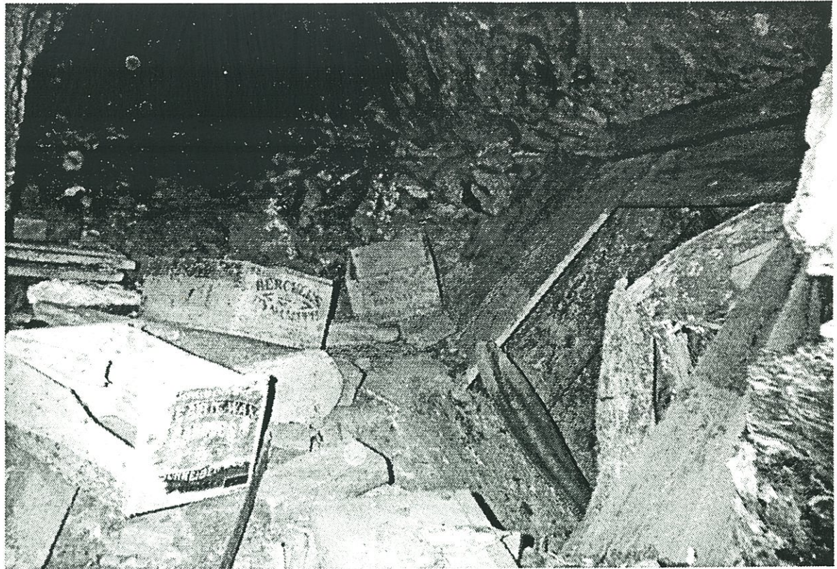
Fallen debris and boxes litter an underground tunnel.
