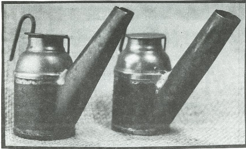
Figure 3. Oil wick lamps by Hunt & Connell (left) and Quinn & Murray (right) both of Scranton.
