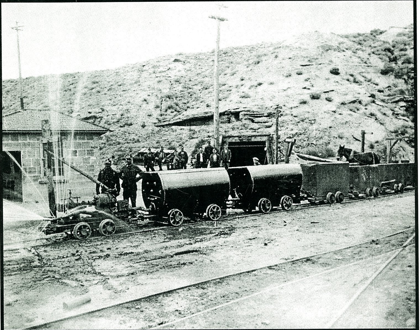
Mine Water Spraying Car
