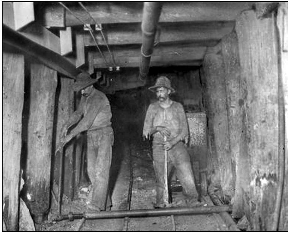
Mine insulators carrying wires in the Speculator mine, Butte, Montana. Dave Johnson collection.
