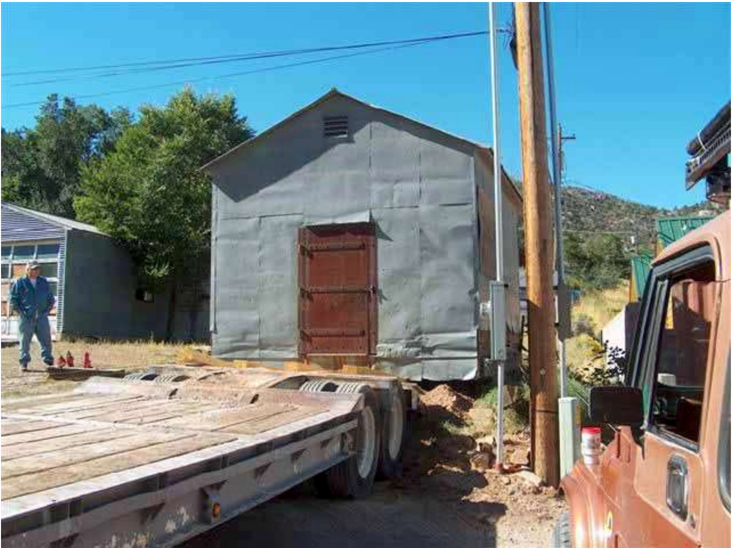
The large flat-bed is backed into position.
