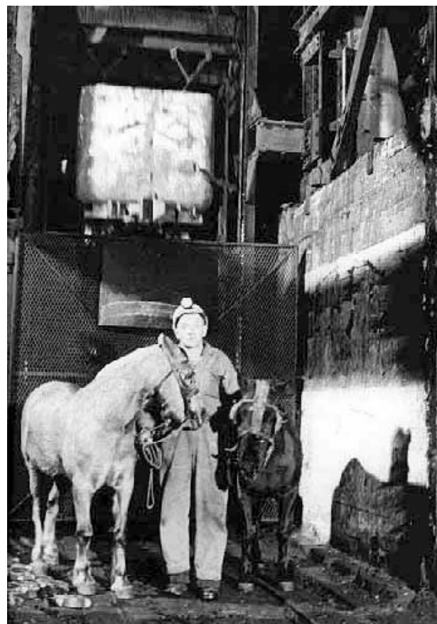
Pit ponies at the hoist cage.
