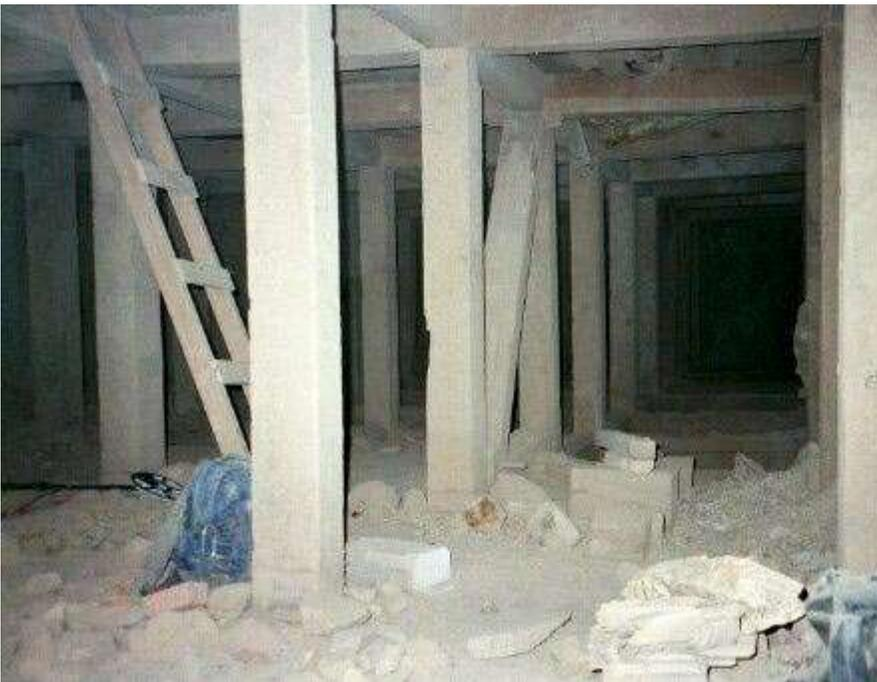
*This is a view from the bottom of the sets looking from the west. You enter the square sets from the west on the next level up. From the bottom there are six levels above. The ladder you see is loose and could be moved around and the miners laid 2x12 planks down to work on.*
