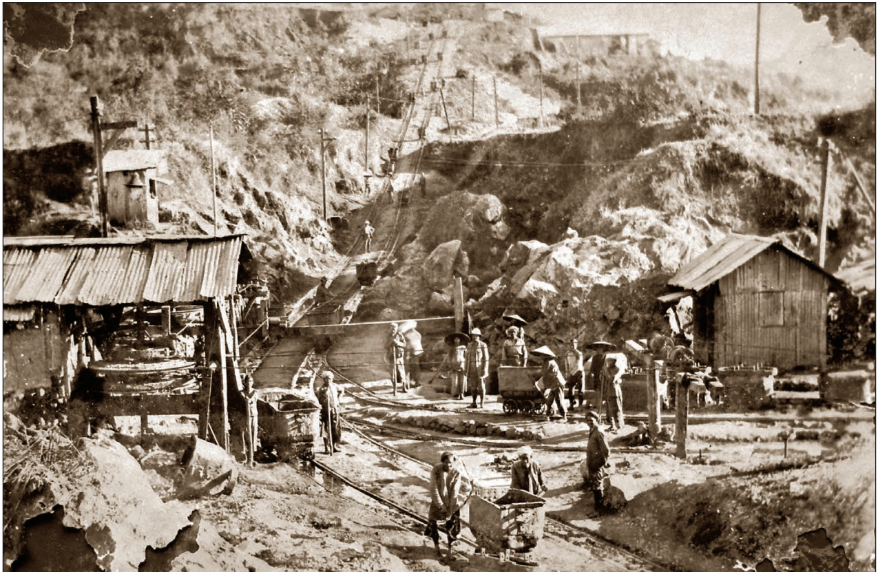
Figure 17. Engine station for ore being trammed down the mountain from ruby workings near Mogok, ca. 1901. Note the double set of rails, one for filled ore cars coming down and one for empty cars going up. Private collection.
